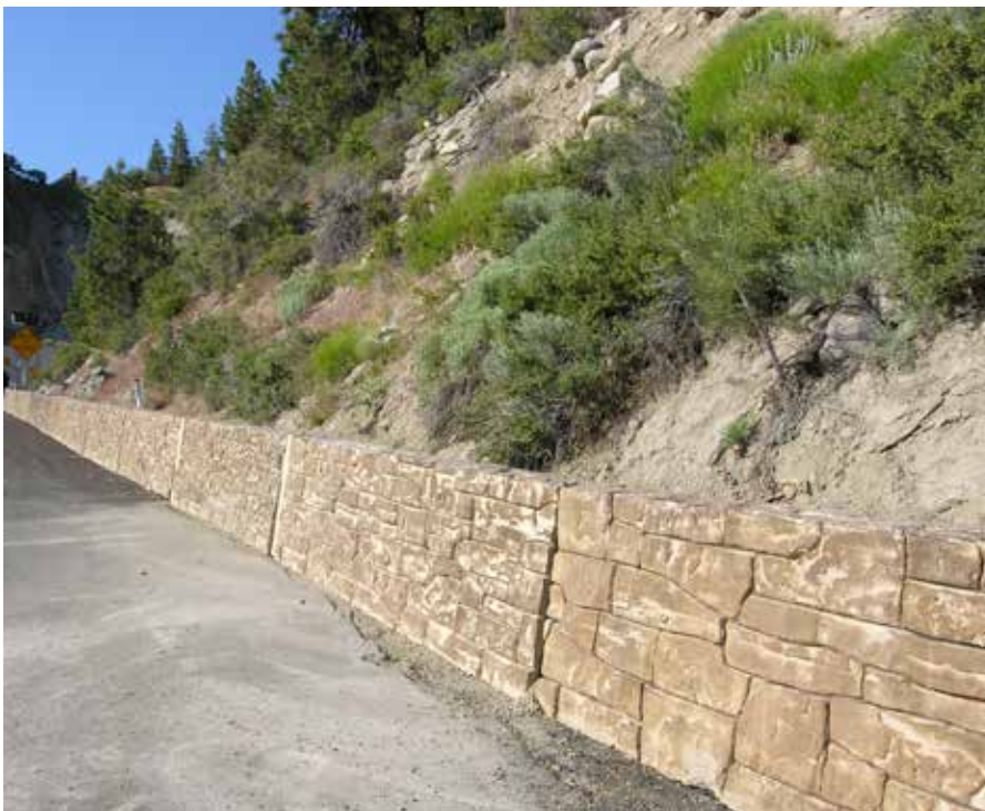
Colors and simple patterning of walls and barrier rails should be the standard in areas of national significance.
