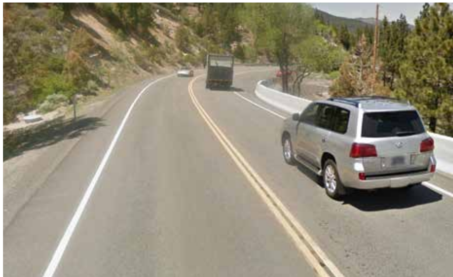
Emergency pull-off locations should be identified every one to two miles through the switchbacks east of Slide Mountain Road.
